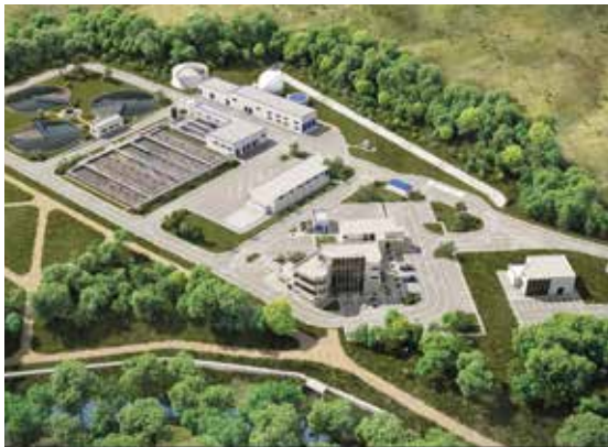
Wastewater treatment plant of Arraiján Est / Panama
