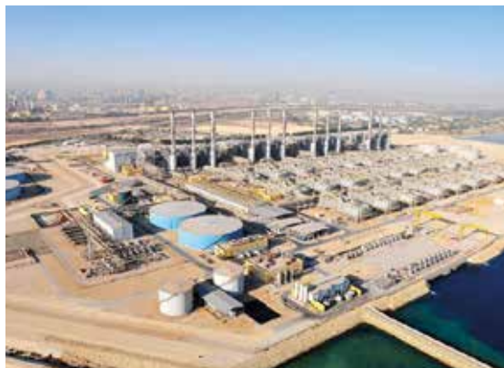
Seawater desalination plant in Les Mamelles, Dakar / Senegal
