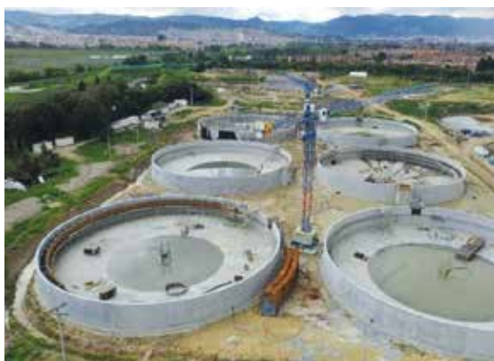
Extension of the El Salitre wastewater treatment plant in Bogotá / Colombia
