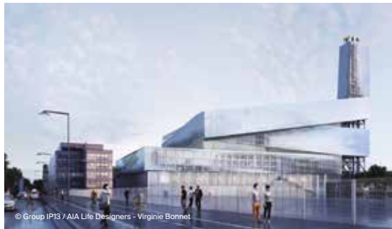
Ivry-Paris XIII waste recovery centre
