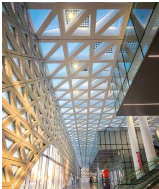
New Kénitra train station
