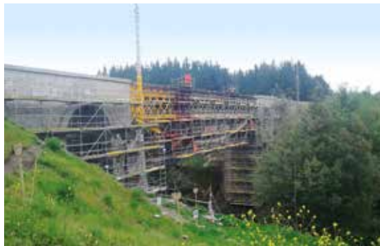
← Rehabilitation and strengthening of a Group 2 bridge
