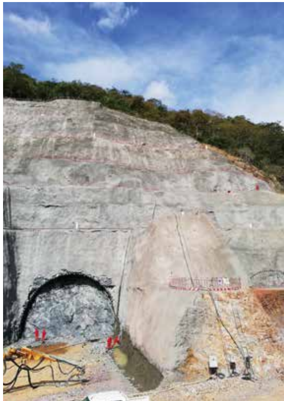
Caculo Cabaça hydroelectric project
