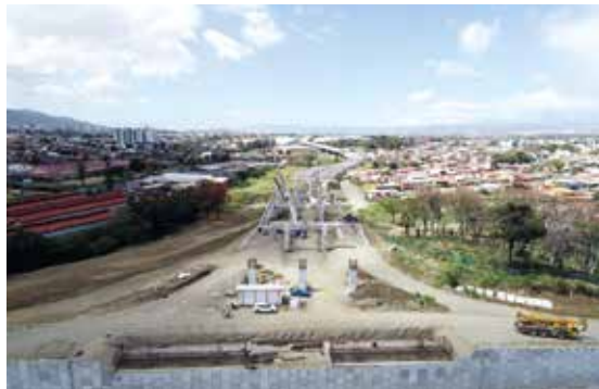
Viaduct – North ring road of San José
