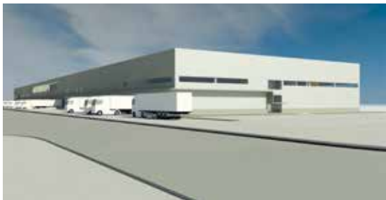
Warehouse for the storage and distribution of frozen food and the headquarters of the Caprabo group, Barcelona / Spain
