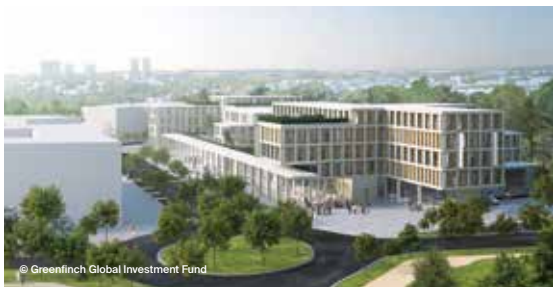
Connection Project, Hamm / Grand-Duchy of Luxembourg
