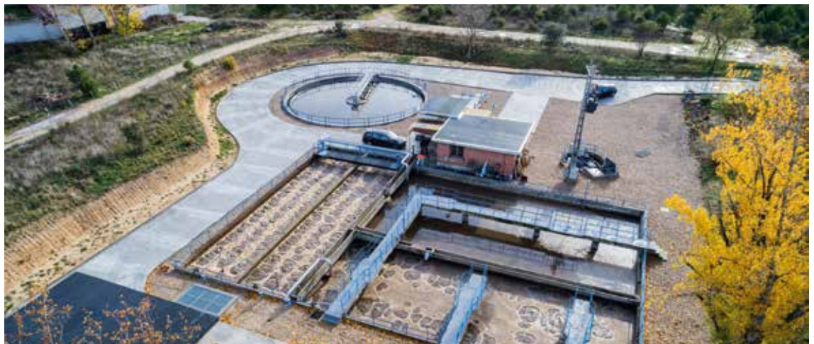
Wastewater treatment plant serving the Autonomous University of Madrid (UAM)
