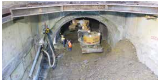
Extension of line 1 of Algiers Metro / Algeria
