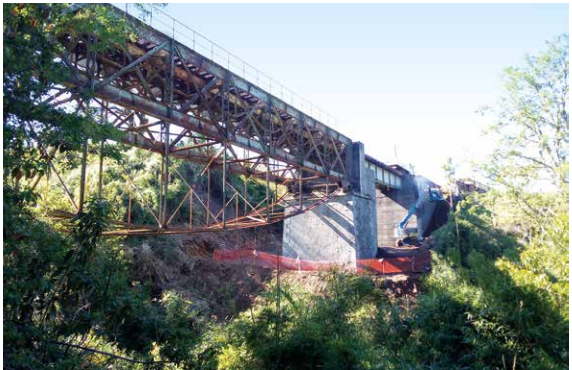
Rehabilitation and strengthening of a Group 5 bridge
