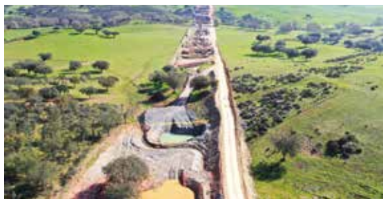
Rail link between Evora and Linha do Esto / Portugal
