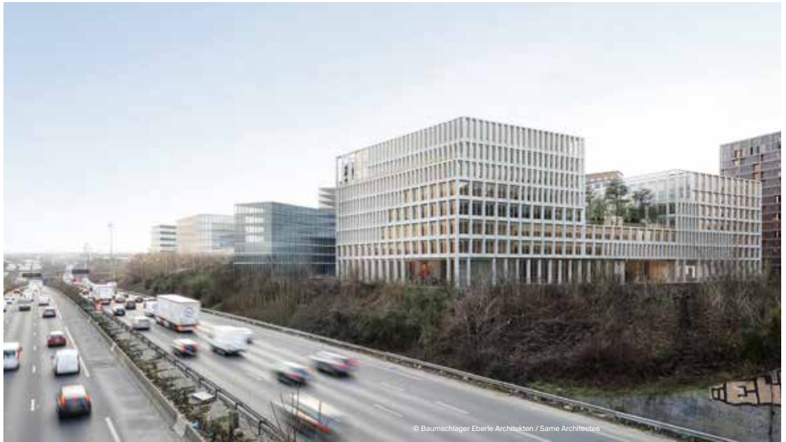
Office building – ZAC Campus Grand Parc
