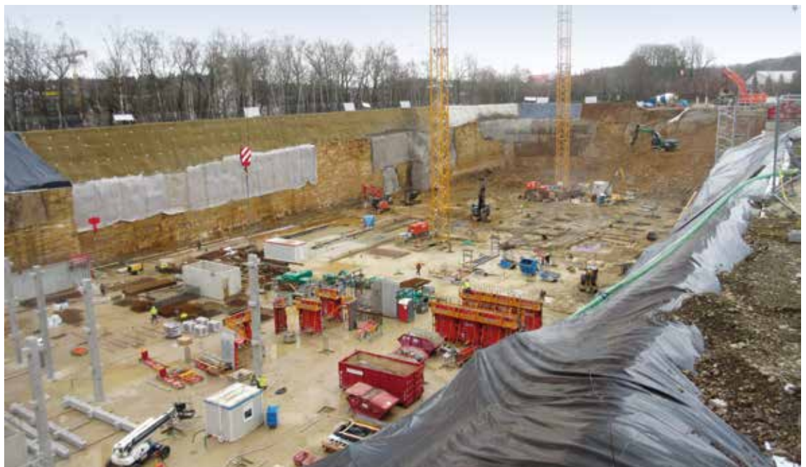
Connection Project, Hamm
