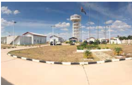
Luena city drinking water distribution network
