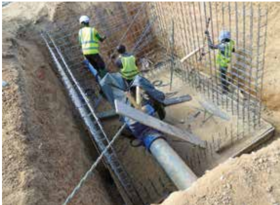
Drinking water supply project for the city of Ouagadougou / Burkina Faso
