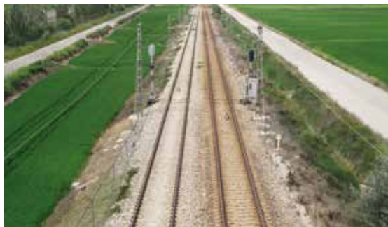
Modernization of the Silla-Cullera section of the line connecting Gandía to Silla
