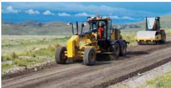
Puno road corridor / Peru
