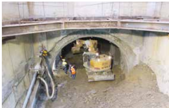
Extension of line 1 of the Algiers metro
