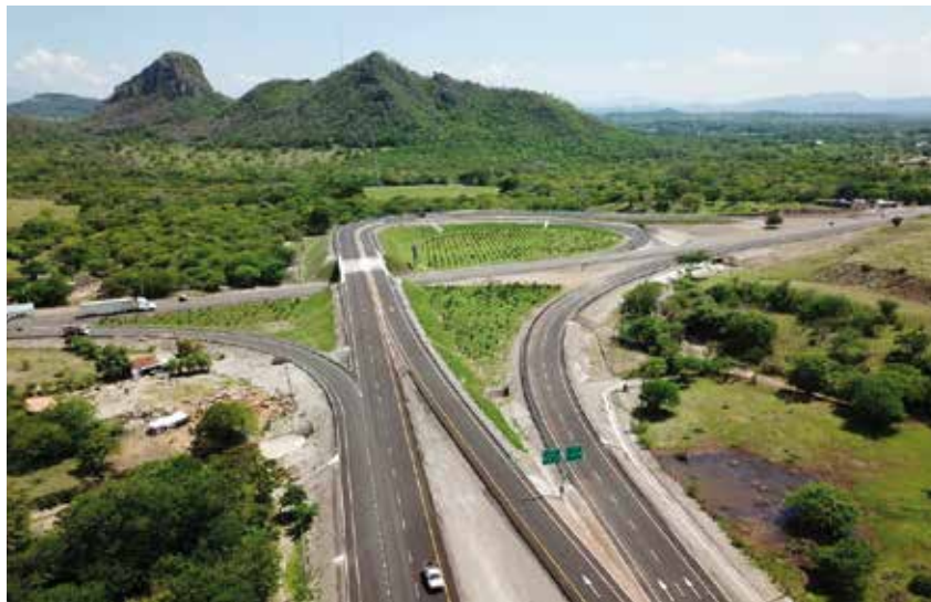
Section III / Corridor logistique Villa San Antonio – Goascoran
